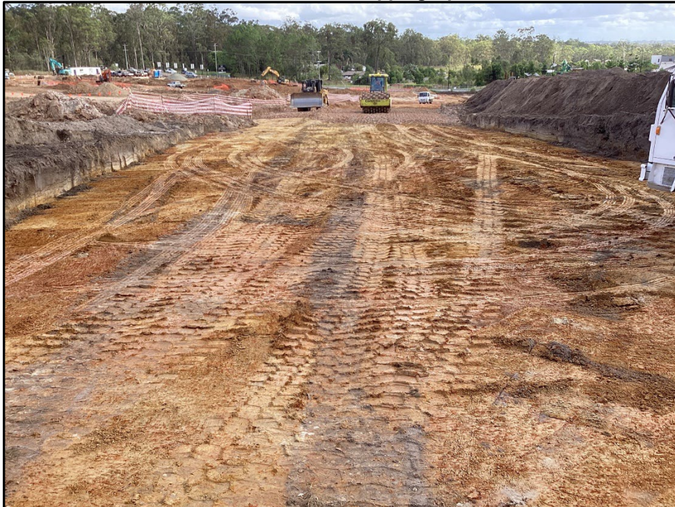
Picture 1: View of the Stripping Operations
