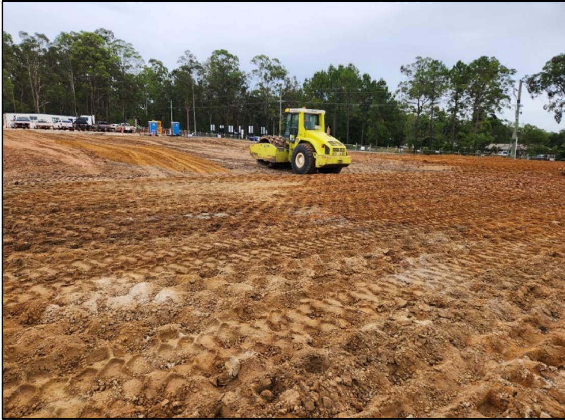
Picture 2: View of Filling Operations
