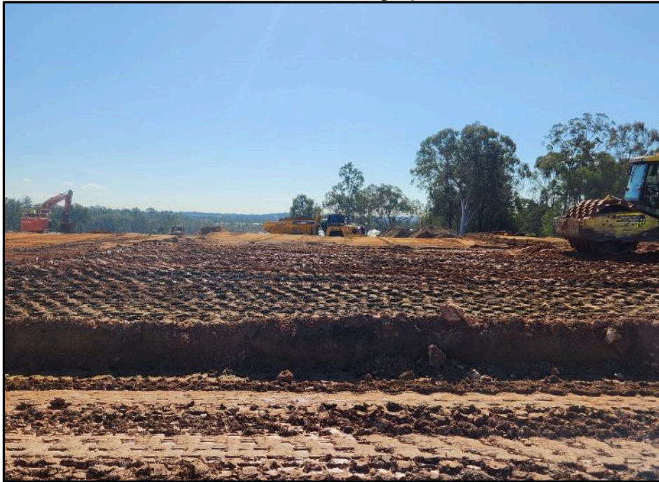
Picture 2: View of Filling Operations
