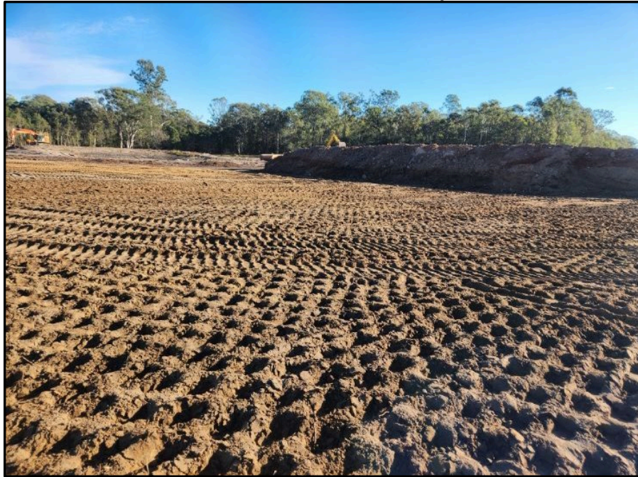
Picture 1: View of Proof Rolled Strip Natural
