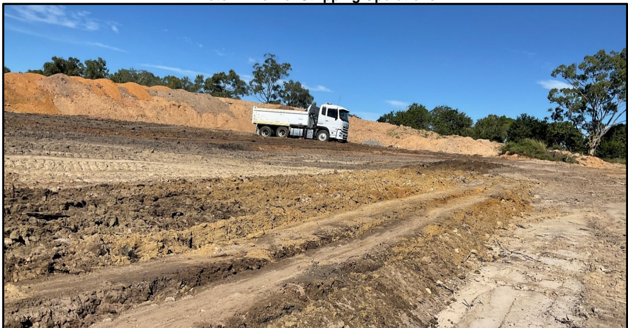
Photo 1: View of Stripping Operations
