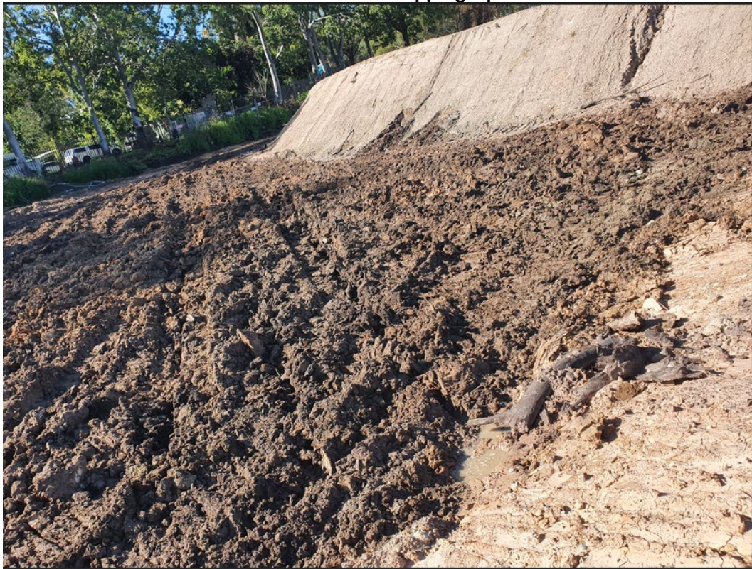
Picture 1: View of the Stripping Operations
