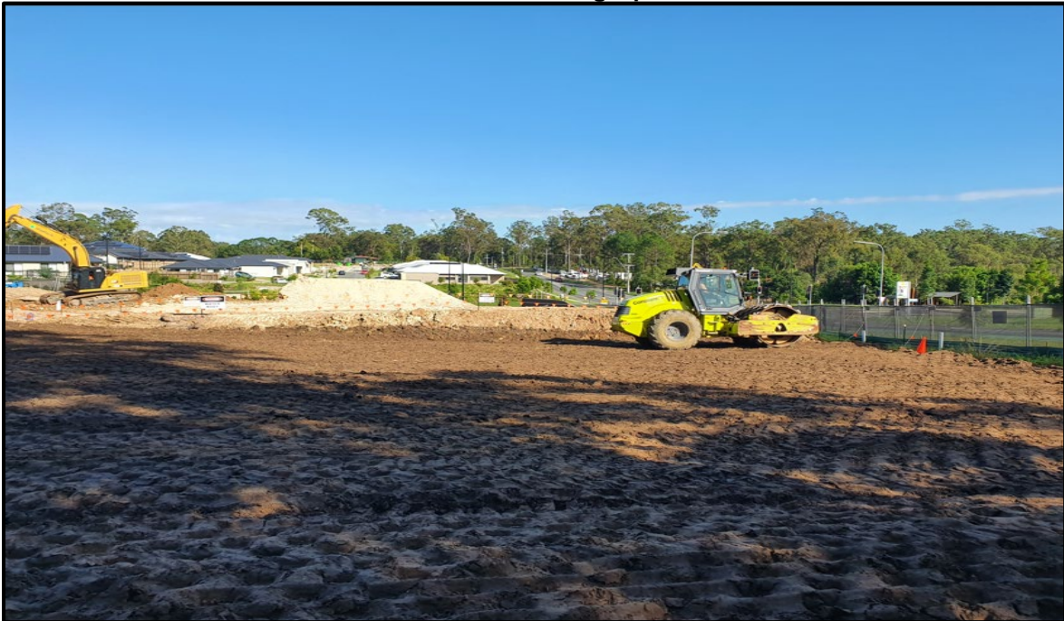
Picture 2: View of Filling Operations
